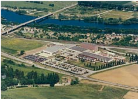
Pont à Mousson (France) is the headquarter of DR FISCHER Europe S.A.S., the production center of infrared halogen and high-voltage lamps.
